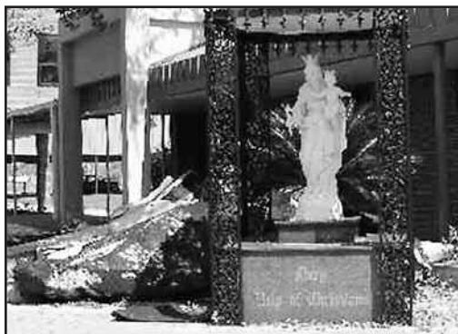
Hurricane Katrina severely damaged St. John Bosco Parish, but the Mary, Help of Christians statue still stands.
